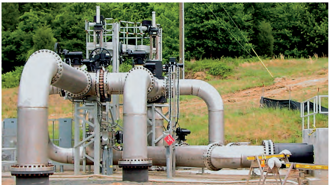
Large diameter 2205 piping installed at the Catawba Nuclear Station.
