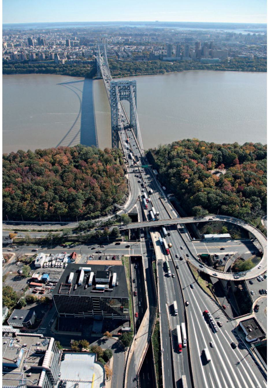
Even though the George Washington Bridge is nearly 90 years old, it adapted to increasing traffic by adding a second deck below the original one in the 1960s, and is now the busiest bridge in the world. © The Port Authority of New York and New Jersey
