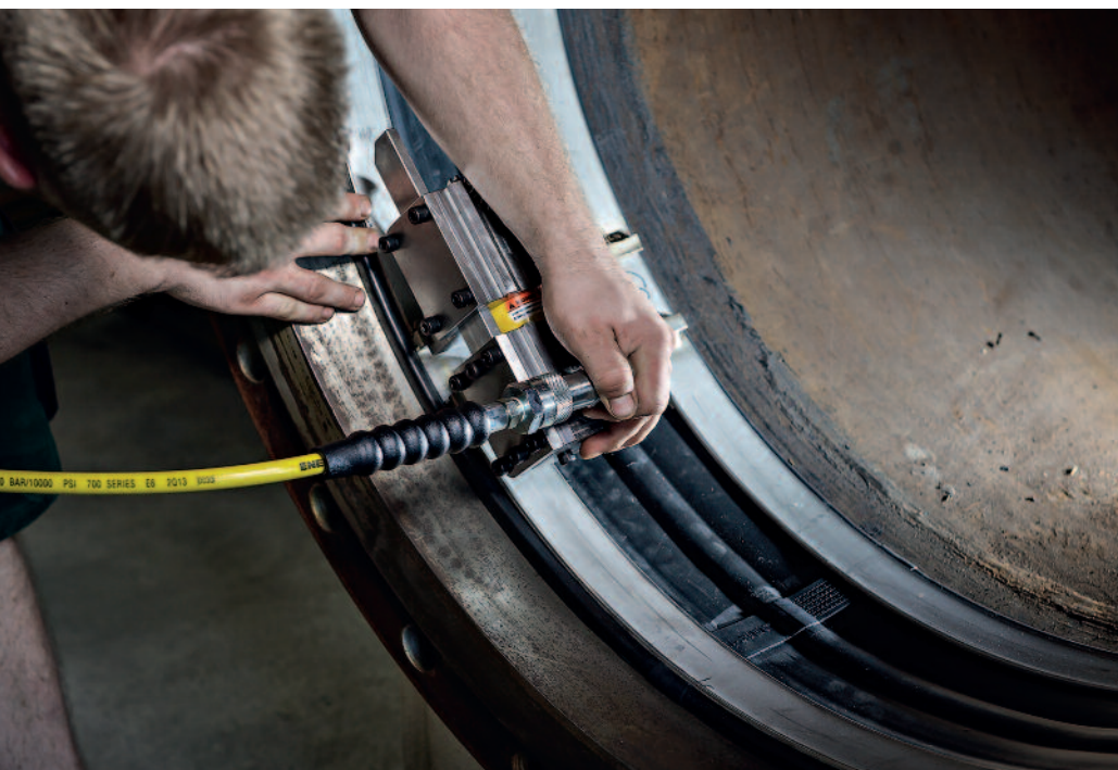
Installation of the internal pipe sealing system. © AMEX
