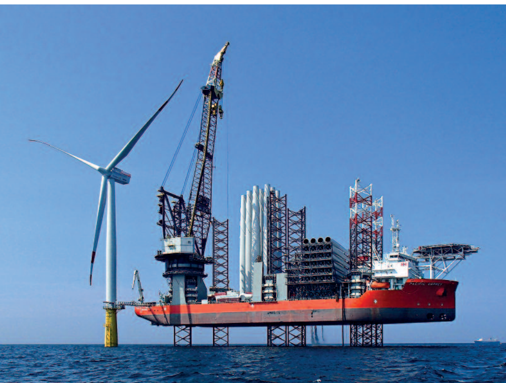
The Pacific Osprey jackup vessel is lifted off the sea and remains stable and disconnected from the waves below for the installation of a wind turbine. © Swire Blue Ocean
