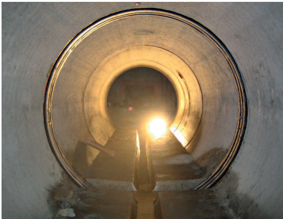
The inside of a large diameter pipe repaired with the sealing system. © AMEX
