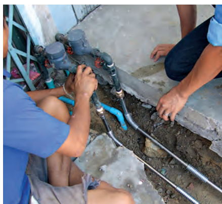
Installation of corrugated Type 316 stainless steel service pipe in Tokyo. © Tokyo Waterworks
