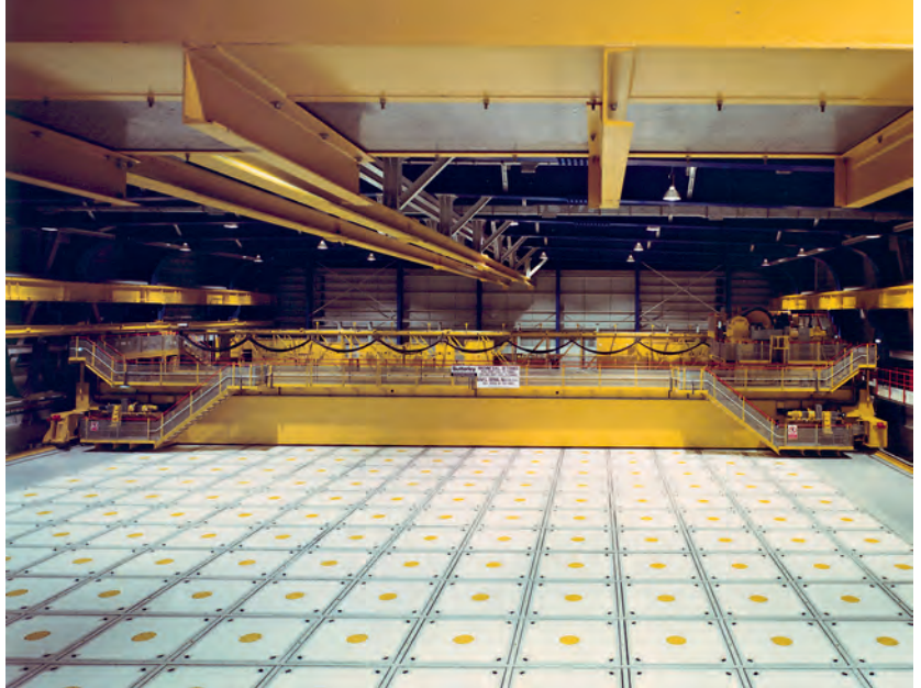
Intermediate level waste drums at Sellafield made from Type 316L stainless steel. The drums are filled with waste and stored in stacks (one stack of ten drums under each white square with the yellow dot) in the Encapsulated Product Store at Sellafield, prior to final geological disposal. © Sellafield Ltd
