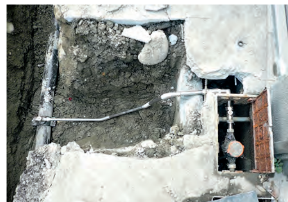
Installation of corrugated Type 316 stainless steel service pipe in Tokyo. © Tokyo Waterworks
