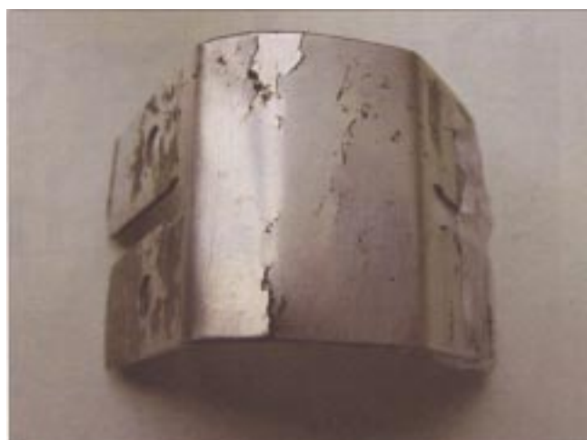
Figure 1: Part of a suspension made of Type 304 damaged by Stress corrosion cracking in the atmosphere of a swimming pool.
