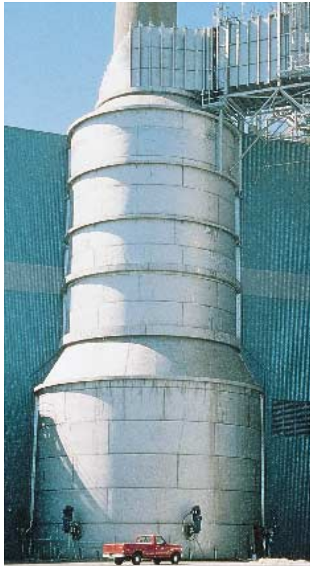
Sulphuric acid plant for the desulphurisation of flue gases
