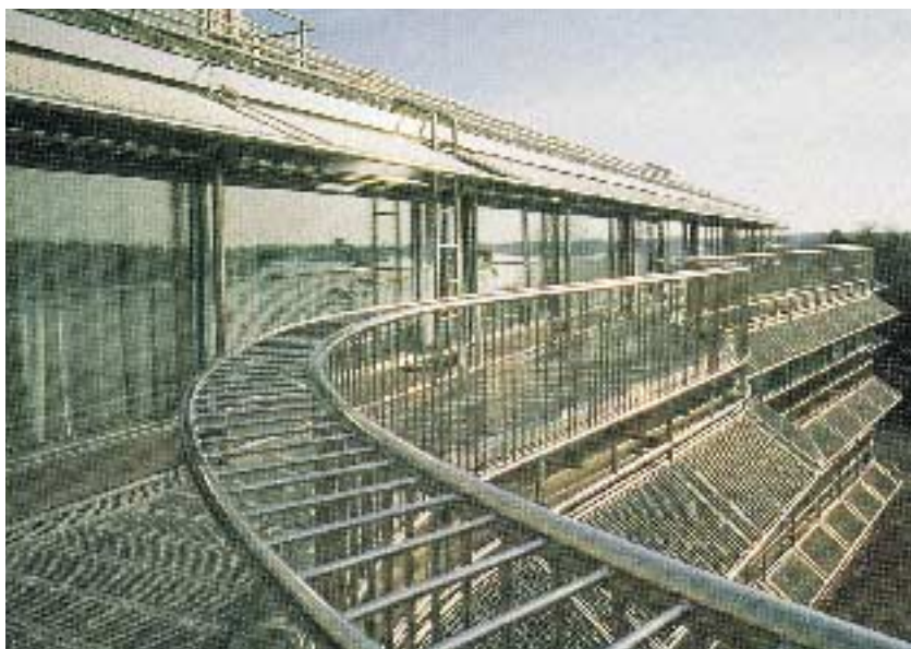
Architectural application of S31600 stainless steel, (2-3% Mo), Finland
