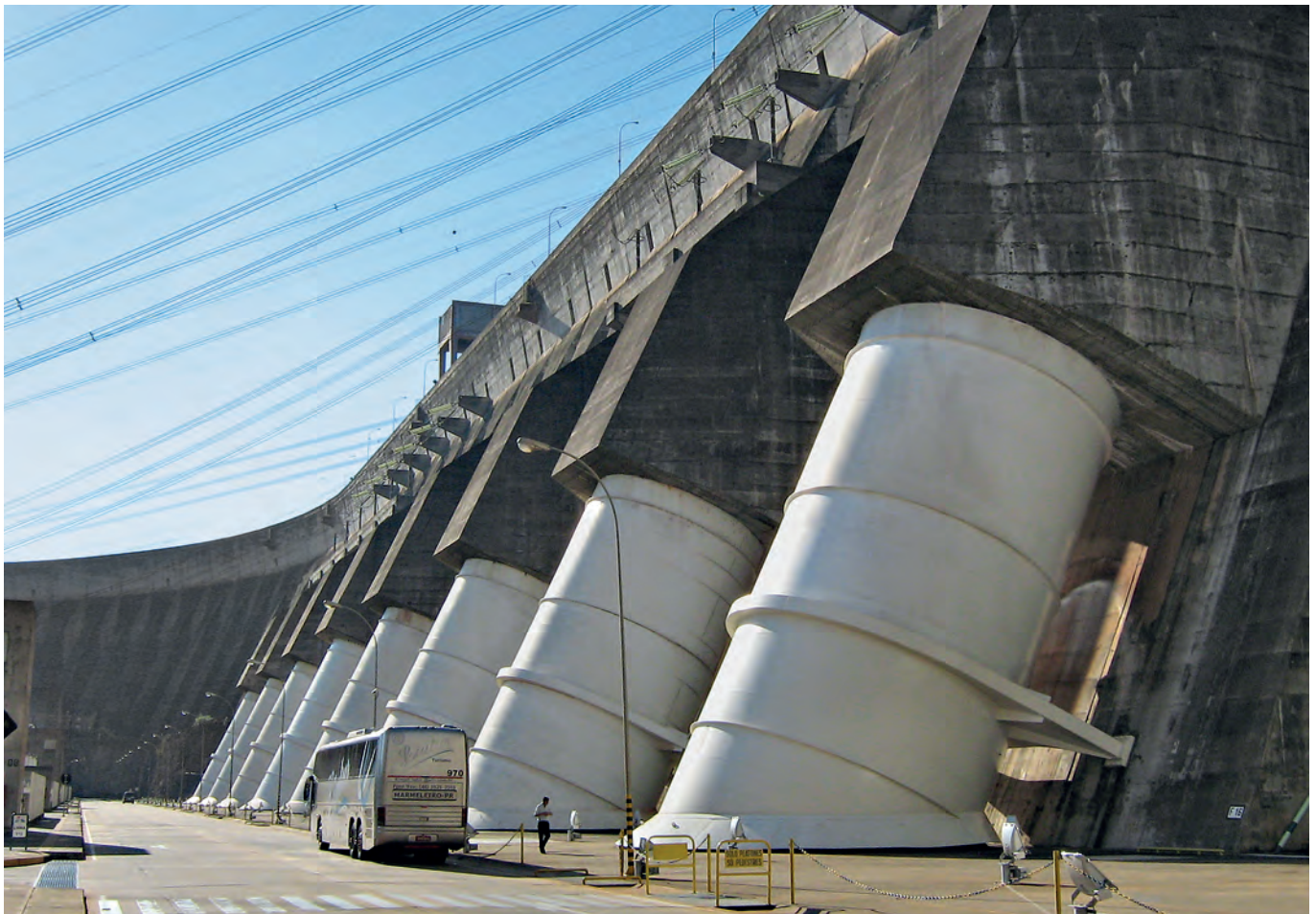
Figure 2. Penstocks of the Itaipú hydroelectric power plant (Brazil/Paraguay).
