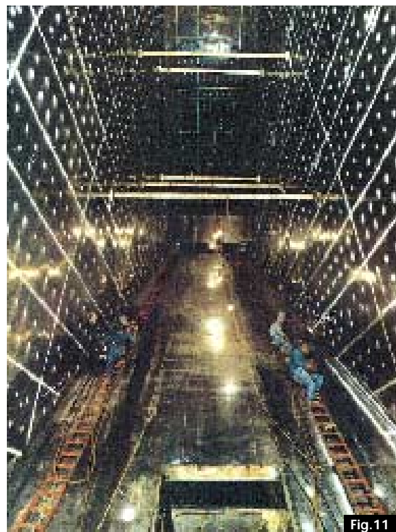
Wallpapered clean gas ductwork leading to the base of a chimney, lined with alloy C-276 (16% molybdenum) to replace failed acid resisting ceramic lining. (Public Service of Indiana, Gibson Power Station, USA)
