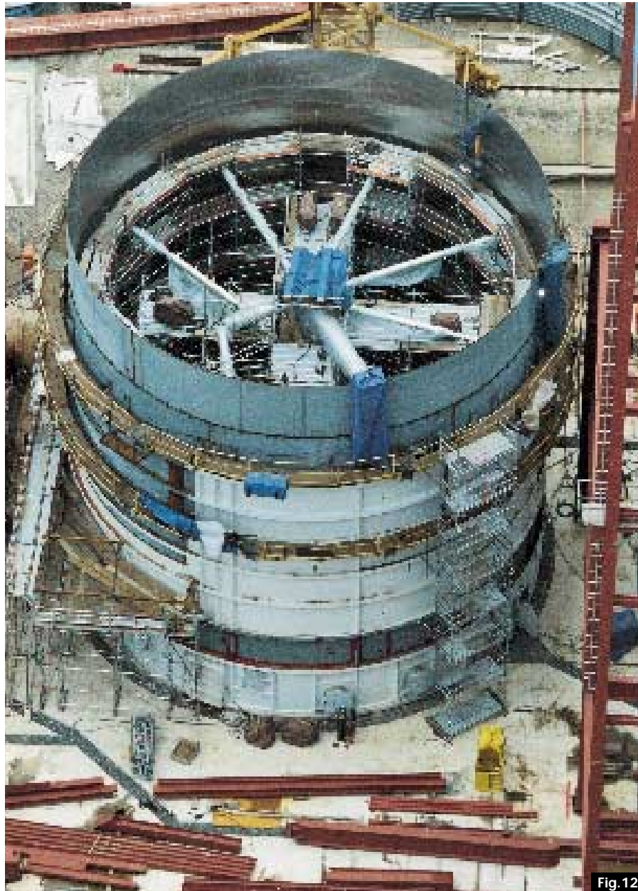
FGD Tower at VEAG power station, Jaenschwalde, Germany. Solid "super" austenitic stainless steel upper section and 16% molybdenum nickel alloy clad plate base, provide excellent corrosion resistance. (Preussag-Noell)
