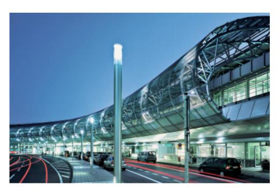
The girders of the hall roof arch elliptically around a 400-metre stretch of the tracks of the new SkyTrain. The outside of the steel and glass construction is clad with stainless steel tubes.
