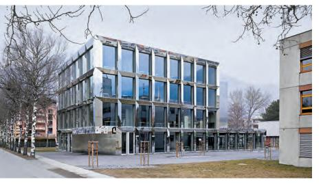
Although conforming to the surrounding development in terms of volume, the new college building is quite different in looks, thanks to the mirror finish of its stainless steel cladding.
