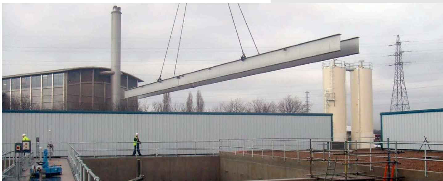
Figure 8: Installation of a pair of main beams
