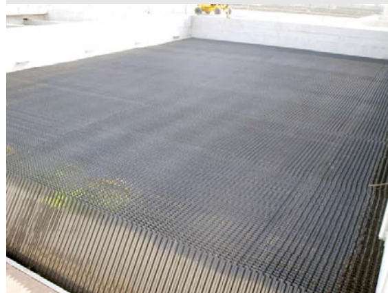
Figure 4: Lamella clarification filter
