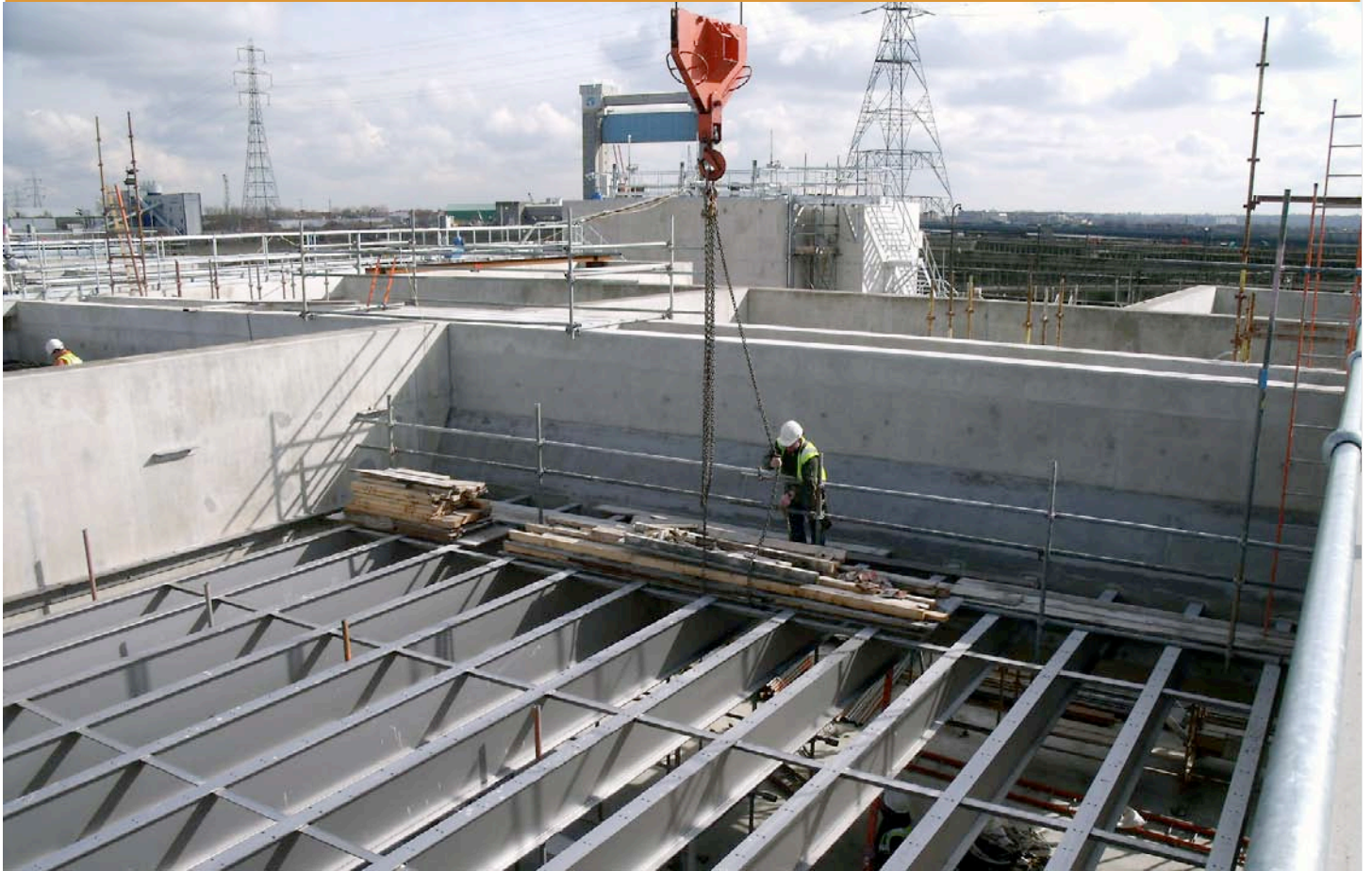
Figure 7: Completed lamella steelwork
