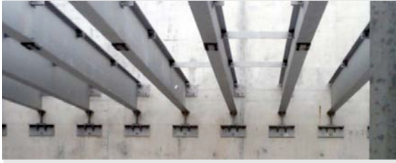
Figure 5: Connection of beams to concrete wall
