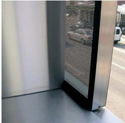
The perforated stainless steel of the sliding panel retains a visual connection with the outside while also protecting against direct sun.
