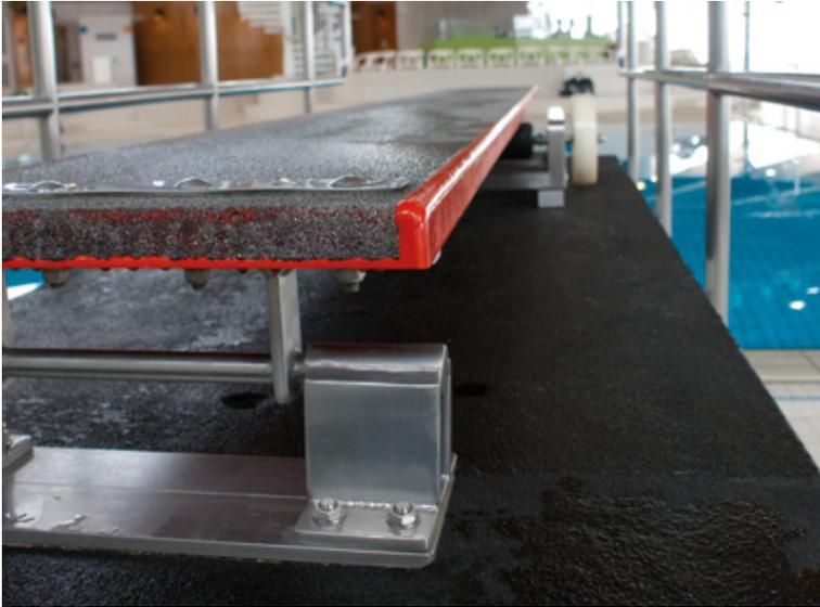
Evaporation, condensation and drying generate a highly corrosive environment in indoor swimming pools. Photo: Fischer, Waldachtal (D)
