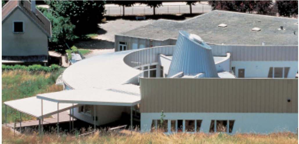
The roofs and the high parapet zones in the façade were clad with the same material – matt-grey stainless steel.
