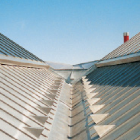
Ventilation caps in the valley gutters take care of ventilation of the roof structure.
