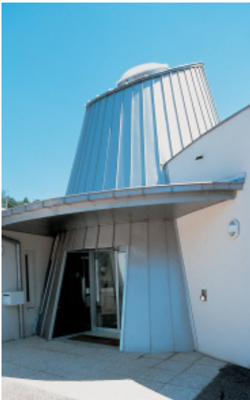
Geometric shapes give a distinctive character to this single-storey complex.
