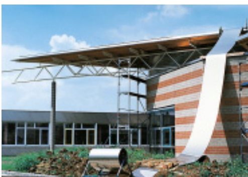
The stainless steel coils are cut to size on site.
