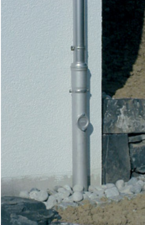
Downpipe with access cover
