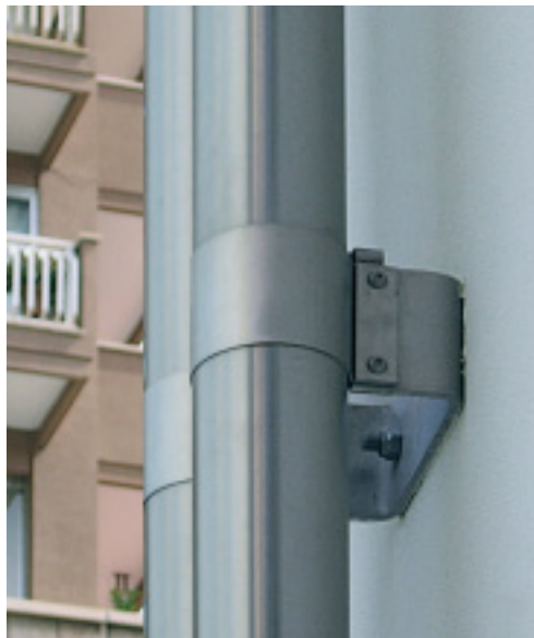
Satin-polished downpipe on the facade of a hotel building at Imperia, Italy
