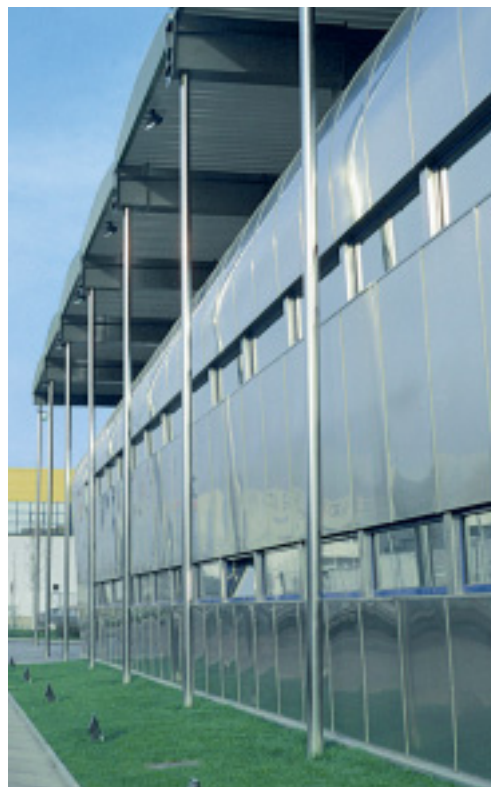
Downpipes made from bright annealed stainless steel at a steel service center at Gavá, Spain
