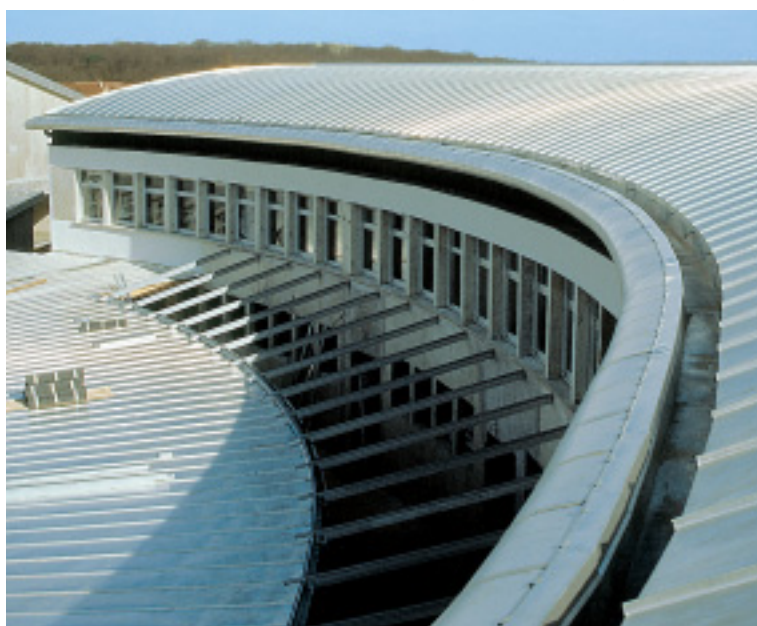
Concealed gutter on a school building at Allonnes, France
