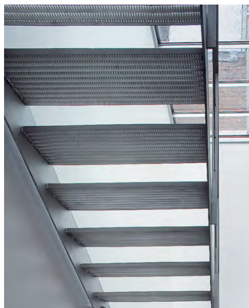
The light, airy style of the interior is continued in the stainless steel handrail profiles and open gridwork treads of the staircases.
