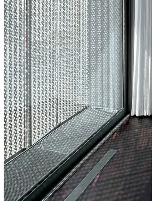
Architectural grating (grade: EN 1.4301) was used for heating vents and for ventilation grilles between the glass panes and the shutters.
