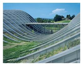
The steel ribs, clad with stainless steel, blend in with the patterns found in the surrounding fields.
