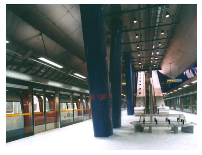
Transport Underground System, all JLE stations have stainless steelframed platform edge doors for reasons of passenger safety and improved station ventilation.
