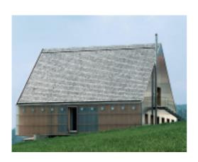
The exhaust gases from the wood-fired central heating system in this detached house are expelled through an external, double-walled chimney of stainless steel. The material itself and the high quality of workmanship ensure many years of trouble-free operation.
