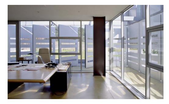
Their exterior walls completely glazed, the offices are equipped with apertured shutters that can be adjusted to optimise interior comfort in terms of brightness and sunlight.
