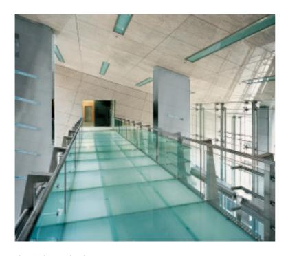
The stainless steel and glass walkway above the main entrance links the two sides of the building at first-floor level.
