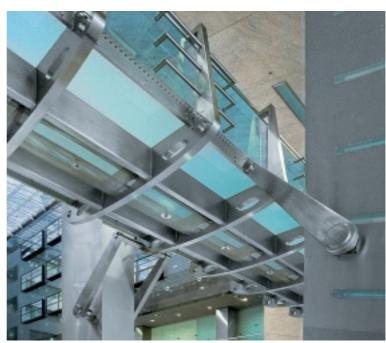
At the mid-point of the walkway loads are directed down into the stainless-steel-clad columns.
