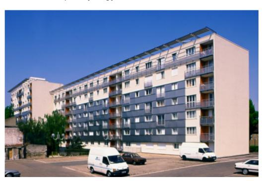
Within the scope of a light rehabilitation operation, this social housing block was given a stainless steel finish over most of its facades.
