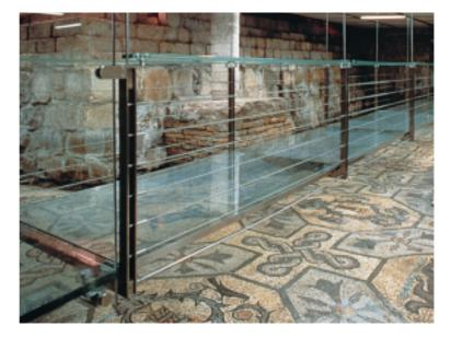
panels prevents any oscillation of the structure. Additional rigidity comes from the tensioning bars spanning horizontally between the uprights either side of the walkway.
