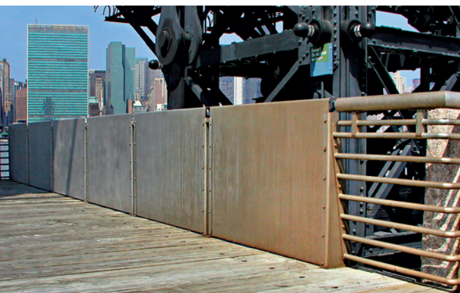
Figure C The Type 316 stainless steel has performed well on the piers. The exception is the splash zone, where there is discoloration caused by corrosion staining (right side of image).
