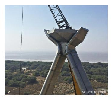
The top of the A-frame during construction, before installation of the glass salt crystal.
