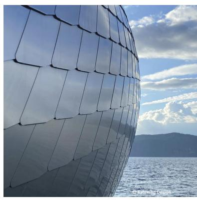
Overlapping shingles that follow the Salmon Eye's elliptical shape brave the harsh environment with minimal upkeep.
