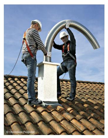
For old chimneys that are not completely straight, a flexible stainless steel liner can follow the required passage.
