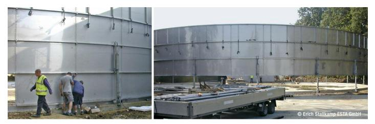
> Two rows of bolts join the prefabricated stainless steel segments vertically. Once an enormous ring is completed, jacks lift it so that the next ring can be assembled at the bottom of the tank. The rings are horizontally connected with special profiles that enhance the stability of the tank wall. All vertical and horizontal joints are sealed.
