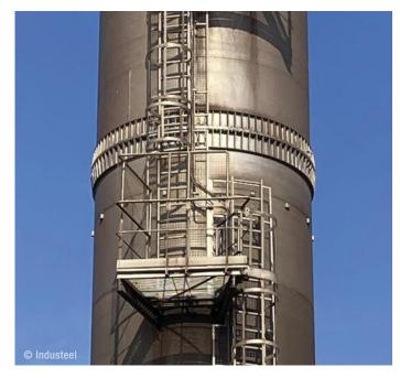
The stack was shipped in segments that were bolted together on site. Ladders and platforms are directly attached to the self-supporting wall. This is much simpler than anchoring them through the outer skin and the thick insulation to the structural inner wall in a double wall system.
