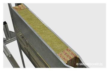
The walls of magnetically shielded rooms consist of layers of mu-metal and aluminum.
