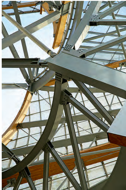
The roof support structure is made of wood, steel and duplex stainless steel components. © Eiffage
