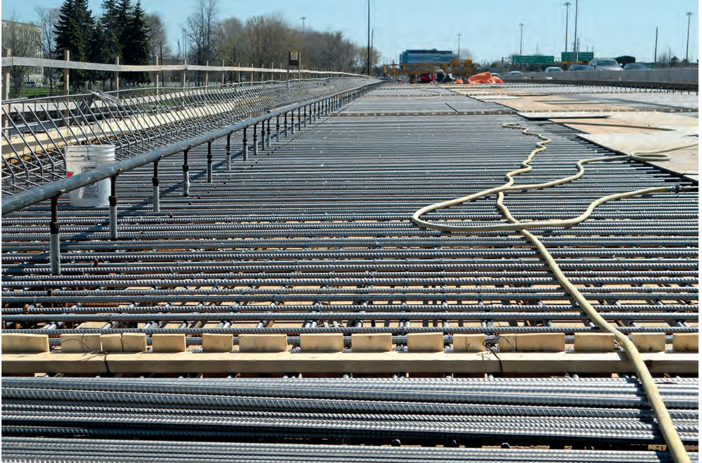
Stainless steel rebar installation on the Hurdman Bridge in Ottawa. The work is done in stages so that some traffic can continue to flow across the bridge as seen in the background of the picture. © Frank Smith
