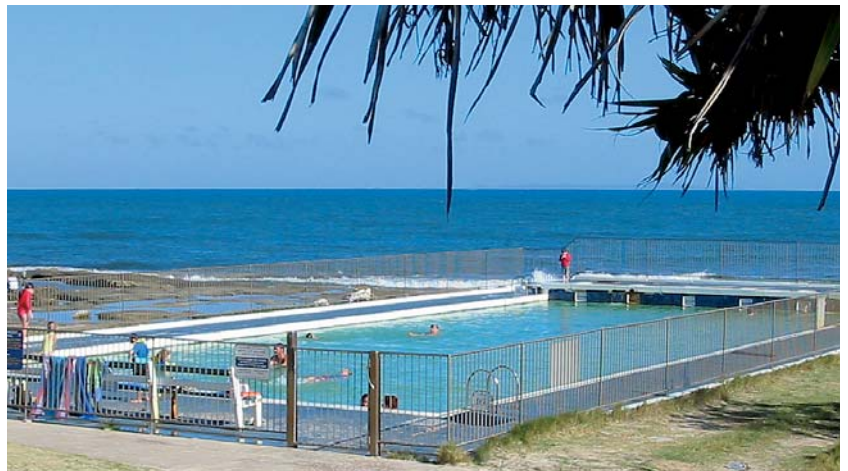
Figure A Stainless steel is used regularly for coastal applications. If properly selected, it can remain attractive and structurally sound in this corrosive environment. (Photo Courtesy of Australian Stainless Steel Development Association)
