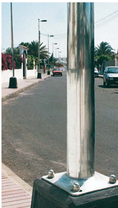
Figure B This shiny Type 316 stainless steel lamppost has been in service for over 10 years. It replaced corroding galvanized steel. (Photo Courtesy of Outokumpu)
