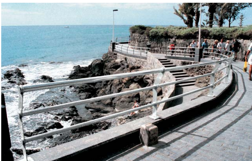
Figure A These 2205 stainless steel railings are exposed to salt spray and occasional splashing. They are in the town of San Augustin in the Canary Islands. There has been no corrosion staining despite exposure to sea spray. (Photo Courtesy of Outokumpu)
