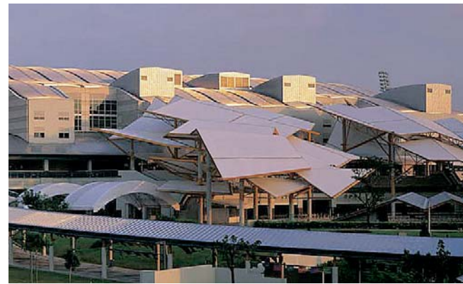
Figure A The Type 316 stainless steel roof of the Singapore Turf Club's grandstand and covered walkway appears to change color during the day. It reflects sunrises, sunsets, blue skies, and clouds. (Photo Courtesy of Ewing Cole, Photographer: Erhard Pfeiffer)
