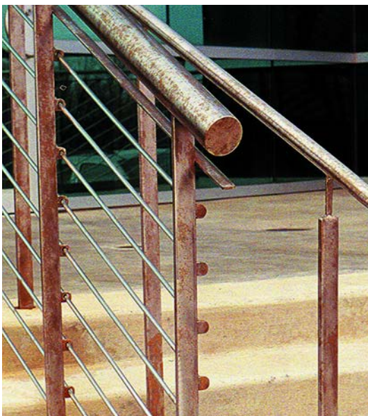
Figure B Type 304 stainless steel with a rough finish was the wrong choice for handrails exposed to deicing salt laden road mist. Cleaning will remove the staining but it will reappear every year. (Photo Courtesy of TMR Stainless)
