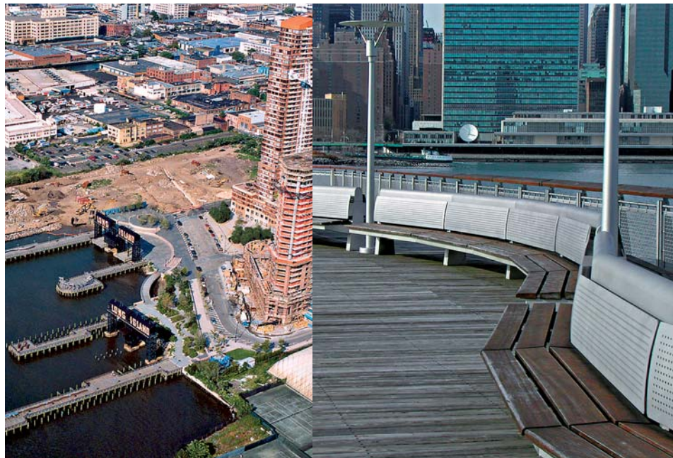
Figures A and B The Gantry Plaza State Park piers jut into the East River and make extensive use of Type 316 stainless steel seating and railings. The United Nations building is visible across the river. (Figure A: Photo Courtesy of Abel Bainnson Butz, LLP)
